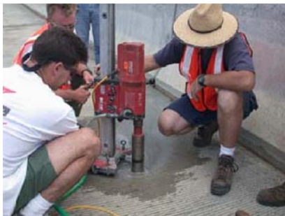
Deck inspection and core sampling.
