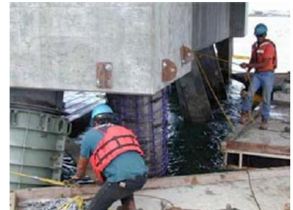
Epoxy coated steel reinforcement.
